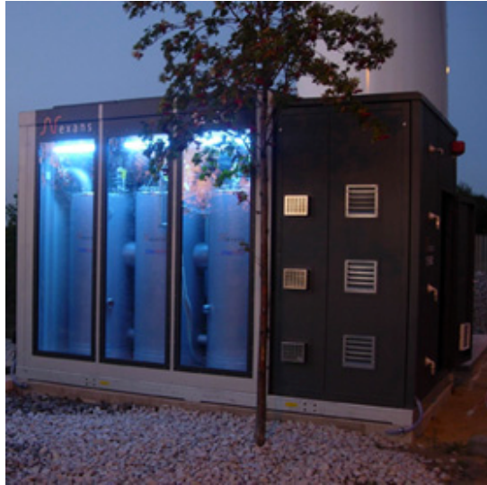
Figure 1.20 – Superconducting Fault Current Limiter from Nexans installed in Germany.
